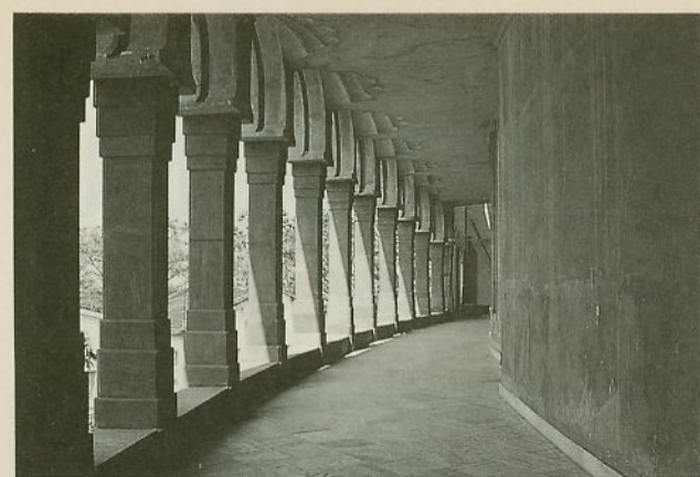
Red sandstone columns line the veranda, which, like most of the building, will be covered in marble.
